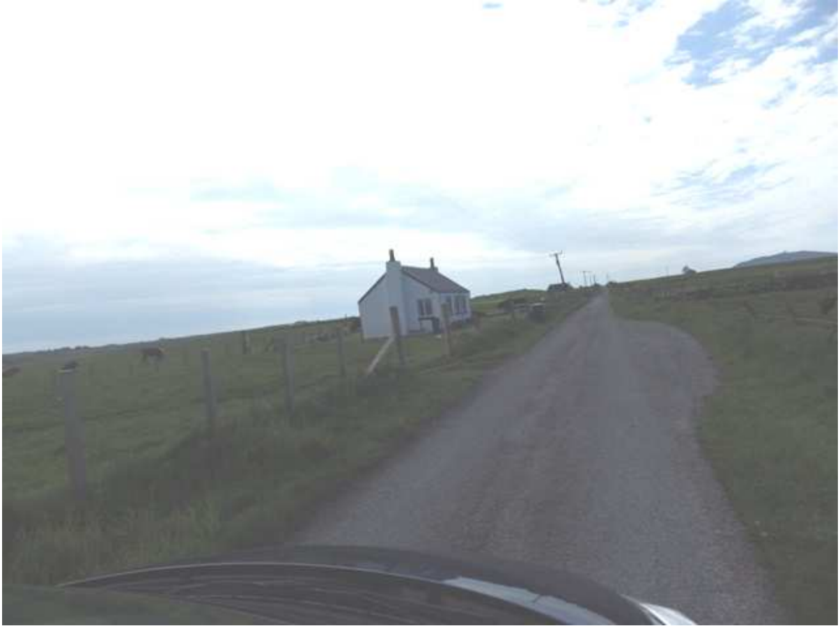
3 – The traditional approach to building in this area is demonstrated down the public road.
