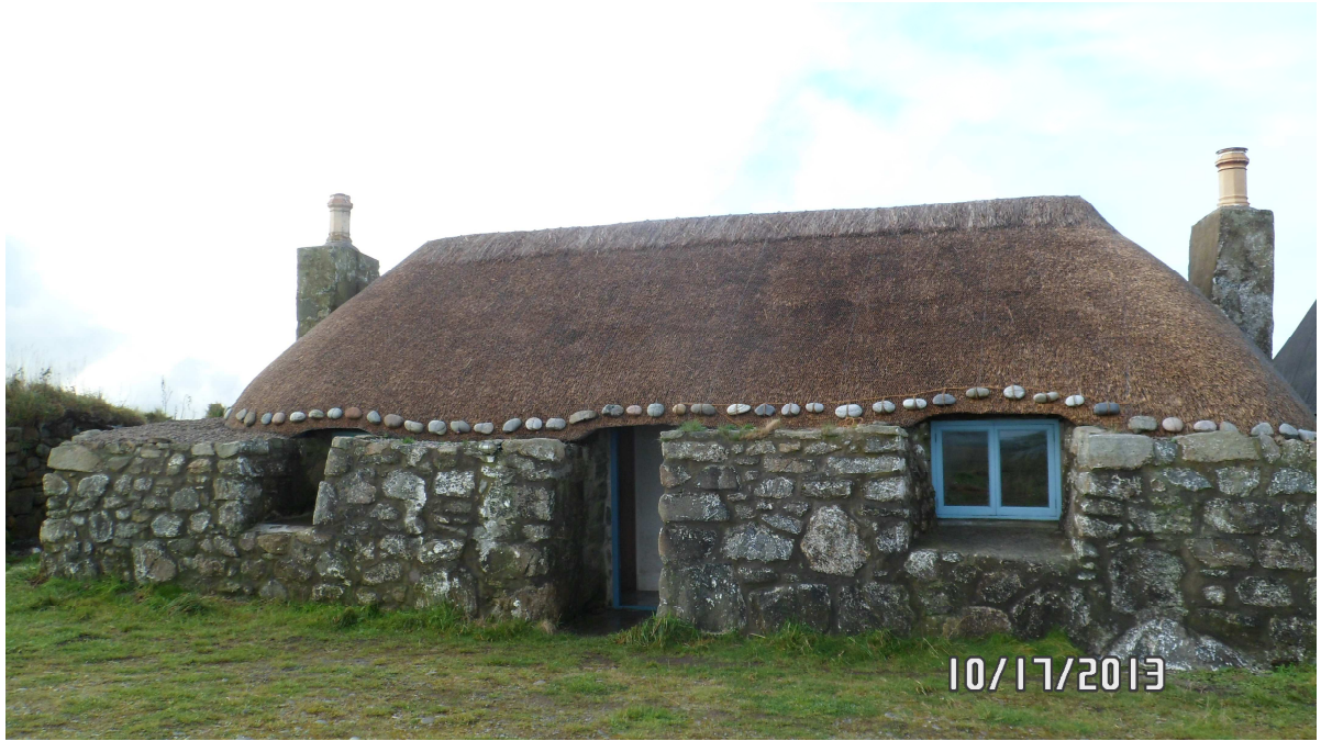
11 – This is the other category A listed building which is located within the conservation area but away from the main road.
